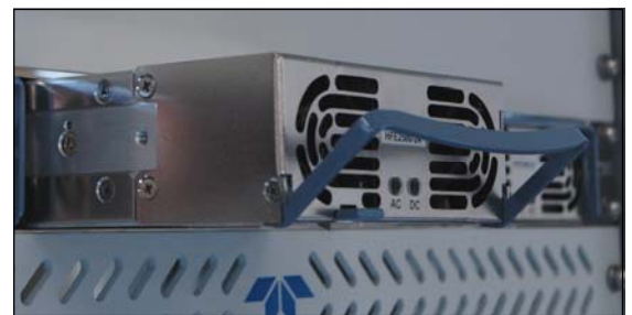
Power Supply Module in Chassis
